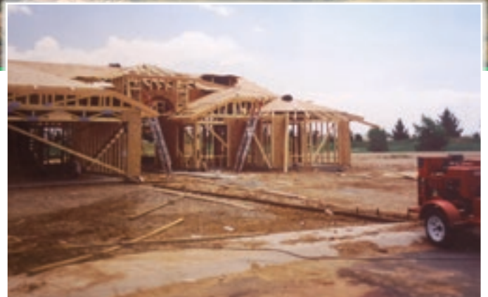
Above: A home is framed out at the Vistas, circa 1994
