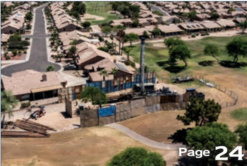
Drilling a well at the Vistas preserves a reliable water source
